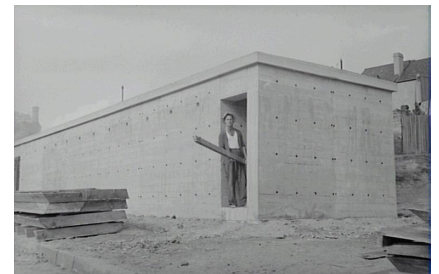
49 Concrete air raid shelter nearing completion.
