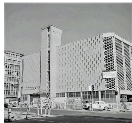
39 The Goulburn Street carpark shortly before completion. The concrete block grilles have since been removed. Source: CSA Unique ID A-00045901.
