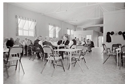
13 Aged Welfare Centre at Newtown in use, February 1959.
