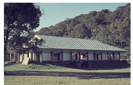
87 The kindergarten at Palm Beach designed by Peter Muller, Source: State Library Victoria ID 1700462, Peter Wille photograph.
