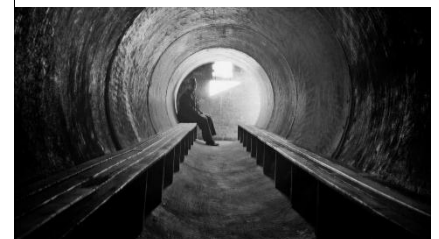
50 Cylindrical air raid shelter.
