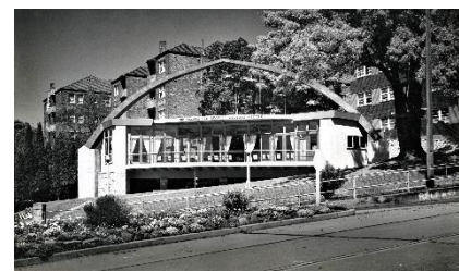
91 Woollahra Old People's Welfare Centre as originally constructed.
