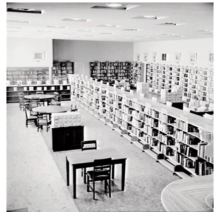
24 Interior of the Frank Green Library at Paddington, November 1952. Source: CSA Unique ID A-00042637.
