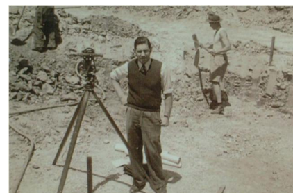
71 Ilmar Berzins on site during the construction of the Arthur McElhone Reserve, circa 1953. Source: reproduced in State Heritage Register nomination for Elizabeth Bay House and Landscape Setting (Arthur McElhone Reserve).
