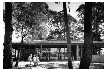
89 The kindergarten at St Ives designed by Collard Clarke & Jackson.
